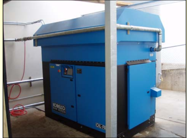
Above: Kobelco KNW Series air cooled oil free compressor with outdoor weather protection.
